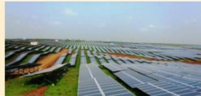
50 MW solar plant in Madhya Pradesh
